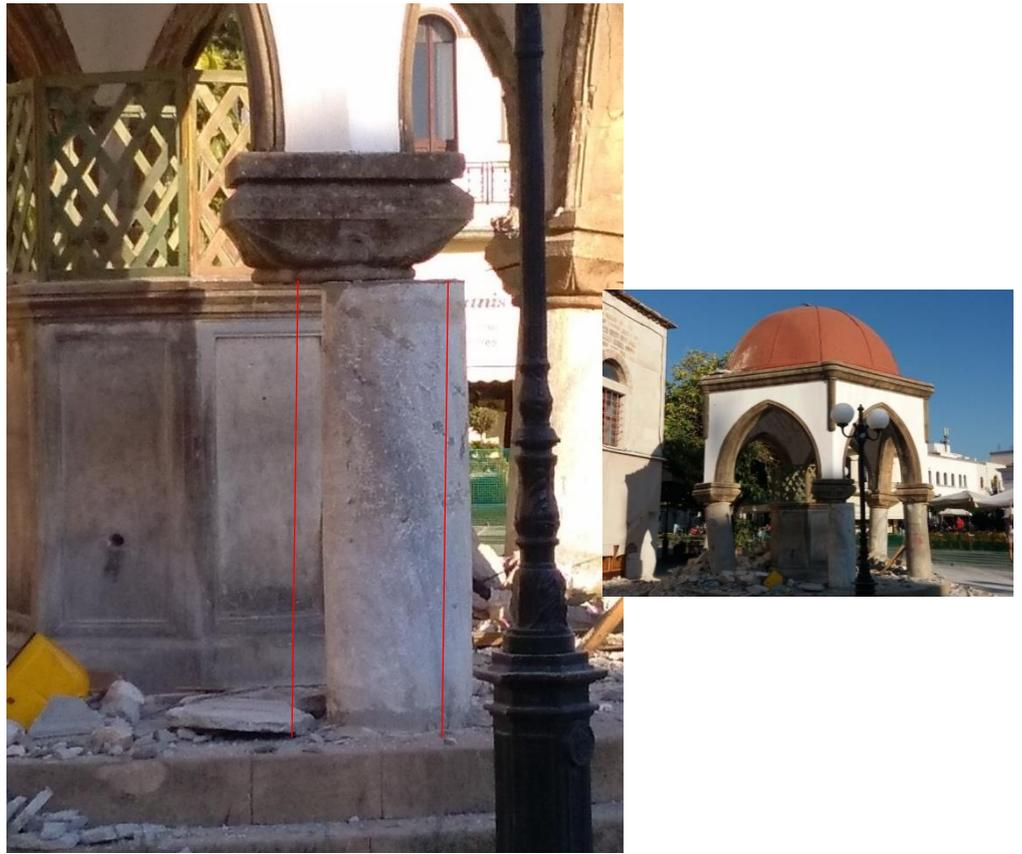
**Figure 7.37: One fountain of Mauritanian style, situated next to the Defterdar Mosque (old part of the Kos city) damaged due to the strong earth shaking but also because the Mosque minaret fell on it. Please note the change of the relative position between the column and the roof structure (red lines).**
