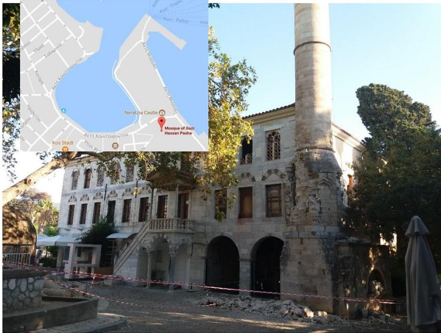
**Figure 7.38: The minaret of the Gazi Hasan Pasha Mosque (old part of the Kos city) was damaged at its base. The Mosque building also damaged.**
